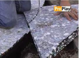
NOTE: when the panels are cut in heated / expanded condition, please cut an extra 1 to 2 cm over the border to compensate for the shrinkage when the ProPlay® cools down
