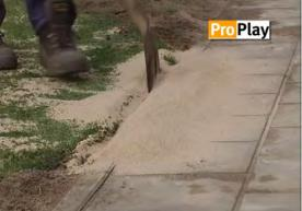
Step 11: Fill the turf with  $25 \text{ kg/m}^2$  sand and spread it evenly
