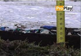
Levelling can be done with a wooden beam, with an edge cut out, and pressing it with a plumb rule; depending on the exact type it is advised to compact the sand
