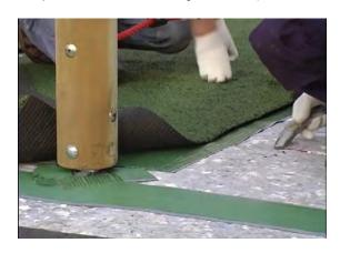
Do not glue the turf (or the synthetic turf tape) on the ProPlay®
