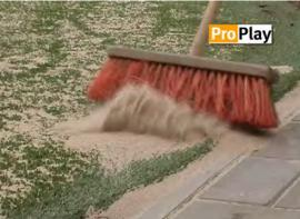
The sand shall be a round 'white' sand, with a grain size of 0.2-1.0 mm
